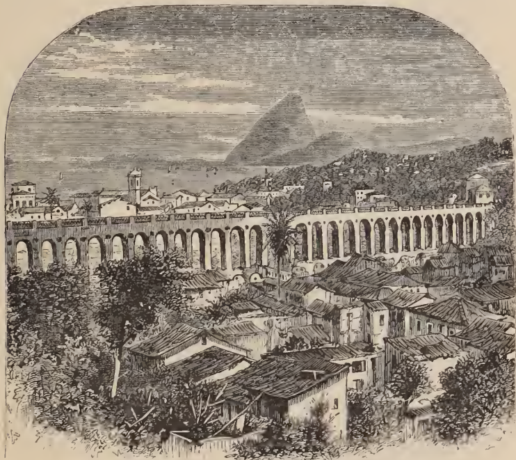
AQUEDUCT AT RIO.
